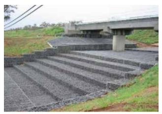
Fig. 1d Bridge Abutment Protection
