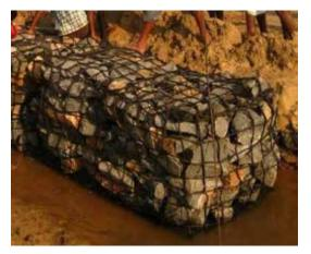
Fig. 3: Polymer Rope Gabions
